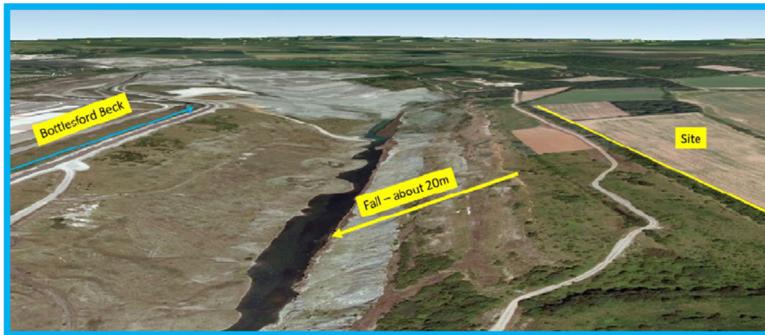
Fig 2 Oblique view of land between the industrial land (British Steel) and the Order Limits, showing the 20m (approx.) deep excavation and standing water (Google Earth image by Getmapping plc).
